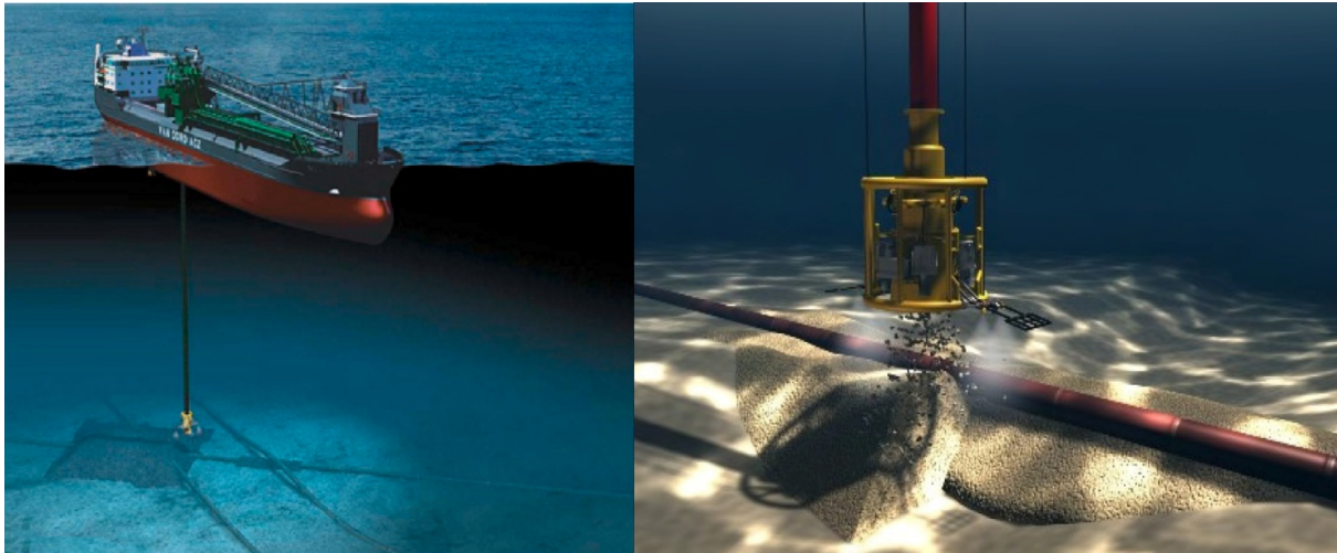
Figure 11: Rock placement on the seabed through a fall-pipe
